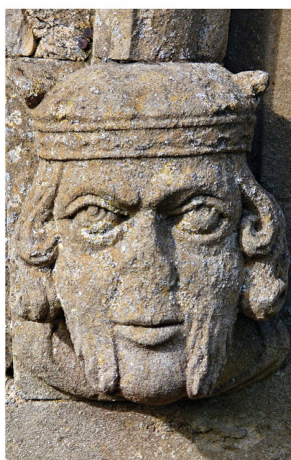
One of two stone corbels by the entrance door
